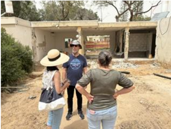
Roni and Ofer are building a new home in Kerem Shalom. Photo: private
